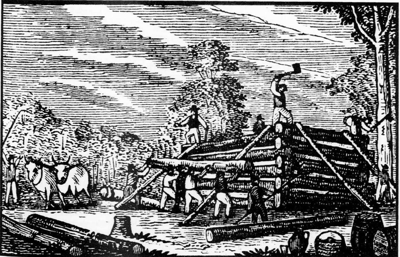
A "RING" OF NEIGHBORS BUILDING A LOG HOUSE IN ONE DAY ROLLING HALF OF A TREE UP A RAMP OF DOUBLE POLES
